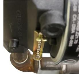
10. Using level chain as a guide, confirm valve is level.
