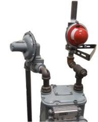
13. **While gas is still off**, open seismic valve. **Do not** open against gas pressure.
