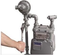
2. Turn gas off at meter inlet valve. **DO NOT** use a pipe wrench.
