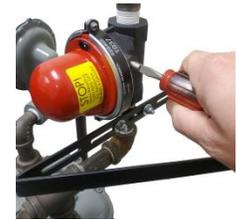
14. Turn gas on at meter inlet valve, **do not** use pipe wrench.
