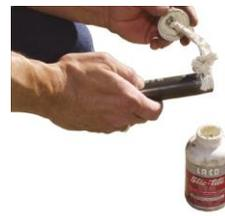
8. Use Teflon tape or liquid sealant on all joints.
