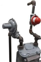
9. Install union gasket and new plumbing from building to meter.
