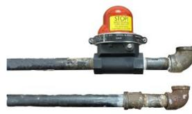
7. Configure new plumbing with PSP valve. Allow 5" to 6" from wall for valve reset shaft clearance.
